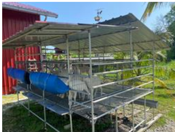
Fig. 4: Goat housing used AA6063-T5 and Galvanized Iron
